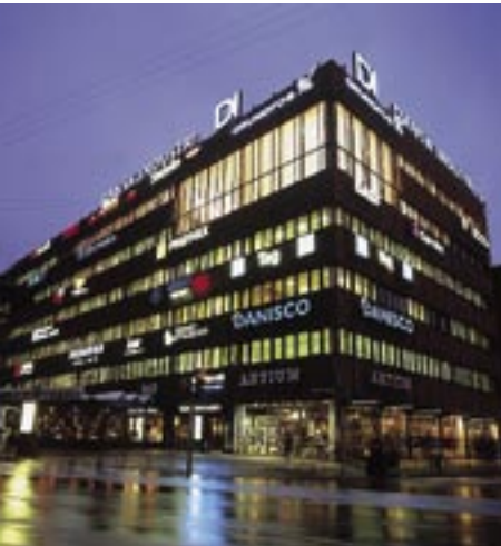
Headquarters of the Confederation of Danish Industries in Copenhagen
