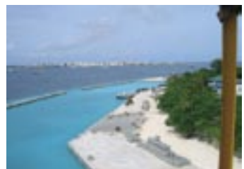
Harbour construction, Maldiv Islands
