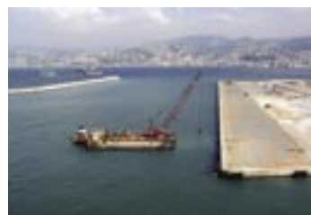
Harbour construction, Lebanon
